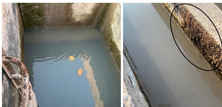
Figure 21. Moo 13's Surface Water Treatment System Contaminated with Leaves and Sediment Accumulated on the Wall (from left to right)
