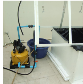
9. Reposition pump and reconnect check valve. Plug pump in, open outlet valve, and run pump for at least 20 minutes to flush old nutrient solution from system. Insure bucket remains full of clean water.
