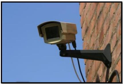
Figure 4: An outdoor CCTV camera with exposed transmission cable
