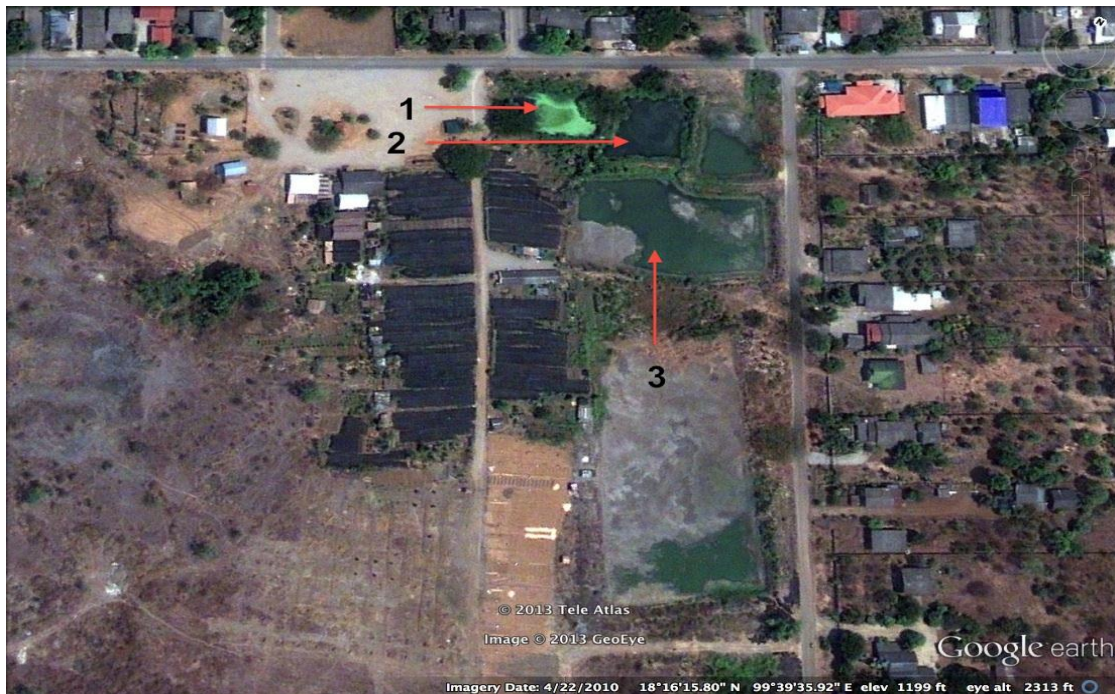
Figure 28: Water purification system at Learning Center based on the Royal Initiative in Mae Mo; pond 1 allows waste to settle while ponds 2 and 3 treat the water
