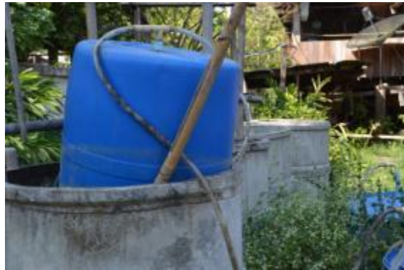
Figure 21: Biogas digester in Chang Nua
