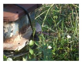
FIGURE 26: EXPOSED WIRES
