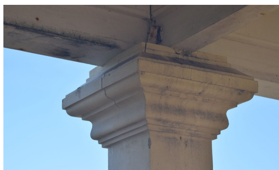
Figure 13. Cracks that form on the special design on top of a column
