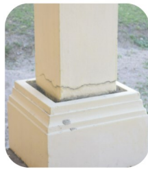
Horizontal Crack
