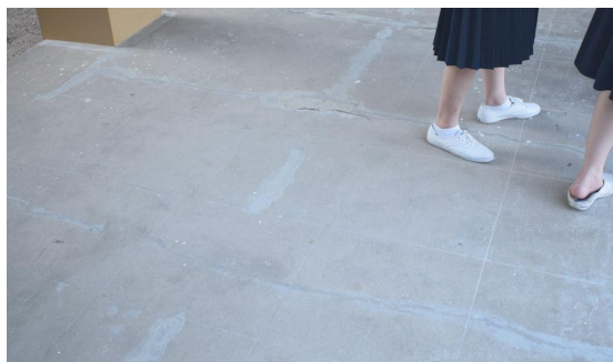
Figure 23. Signs of the difference in concrete colors in the concrete walkways
