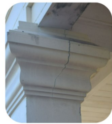
Vertical Crack
