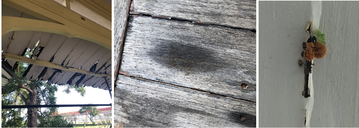
Figure 14. Photos of wet wood and the growth of fungi at Mrigadayavan Palace.
