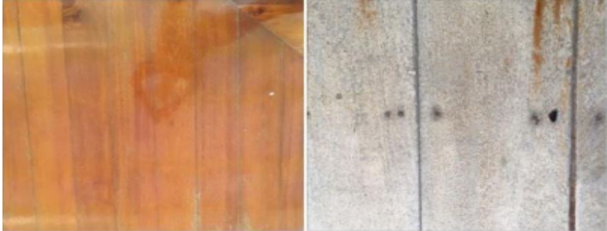
Figure 11. Comparison of original wooden floor (left) and structure after previous restoration (right) of wooden floor. Reprinted from The Restoration Management of Mrigadayavan Palace by Sakunjaroenpornchai, P. (2017).
