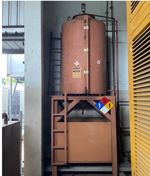
Figure 13: Breather on lubricant and fuel storage
