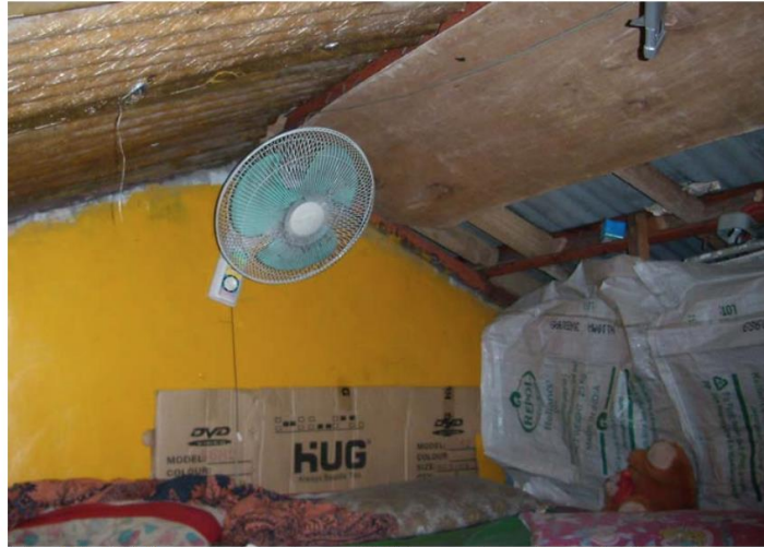
Fig 35. A loft constructed in a GK house shows how dark and cramped it could be. The electrical fan is necessary since there are no windows.
