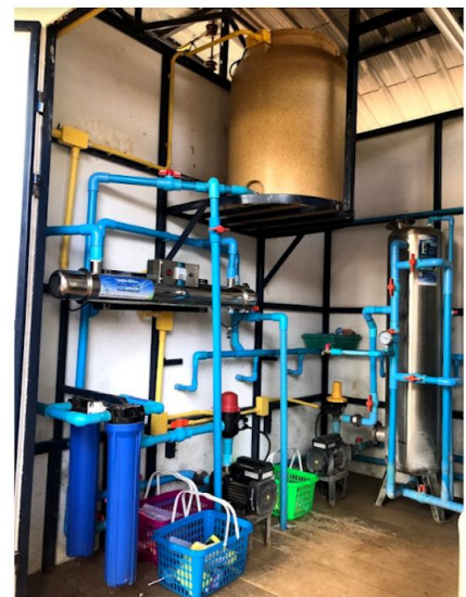
Figure 10. The water filtration systems at Ban Mae Salap including carbon filtration, sand filtration, UF, MF, UV, and RO.
